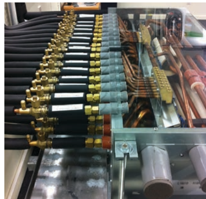
Mitsubishi Electric branch controller fitted with refrigeration ball valves for ease of maintenance and fit out flexibility.
